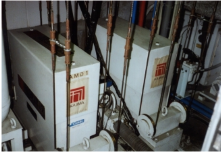
Kyobashi Seiwa Building – Main AMD Masses (4.2 metric tons)
