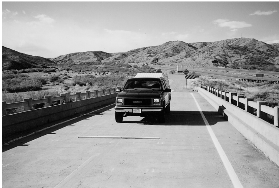
Figure 12 – Forced vibration induced by a speeding truck crossing the bridge
