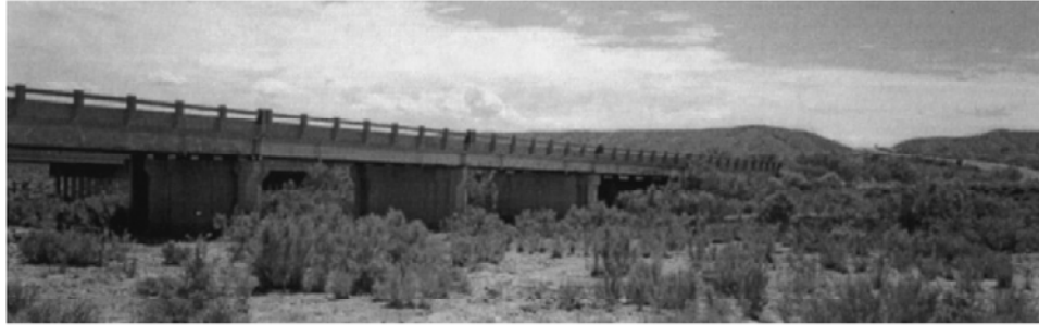
Figure 1. A side view of the Alamosa Canyon Bridge
